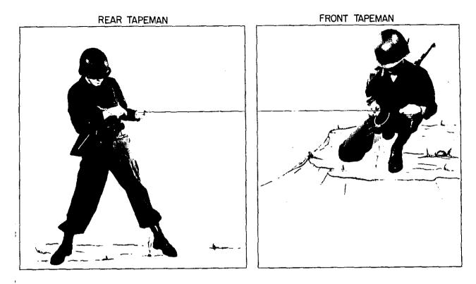
Figure 11. Applying tension to a tape.
